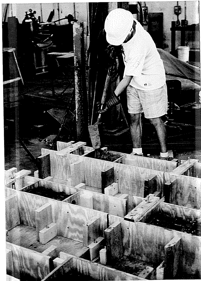
Figure 3.9 Placement of Concrete in Formwork
