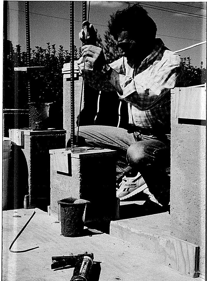
Figure 3.13 Rodding of Non-Shrink Grout
